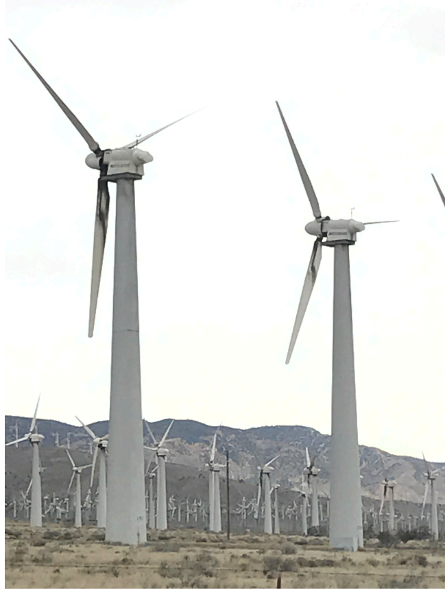
Figure 3: Abandoned, aging infrastructure.
