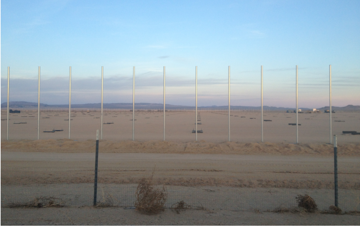
Figure 2: Breaking new ground on SEGS Generation Facilities VIII-IX. No vegetation remains and the area is fenced off. The electricity from this facility will primarily feed Las Vegas.
